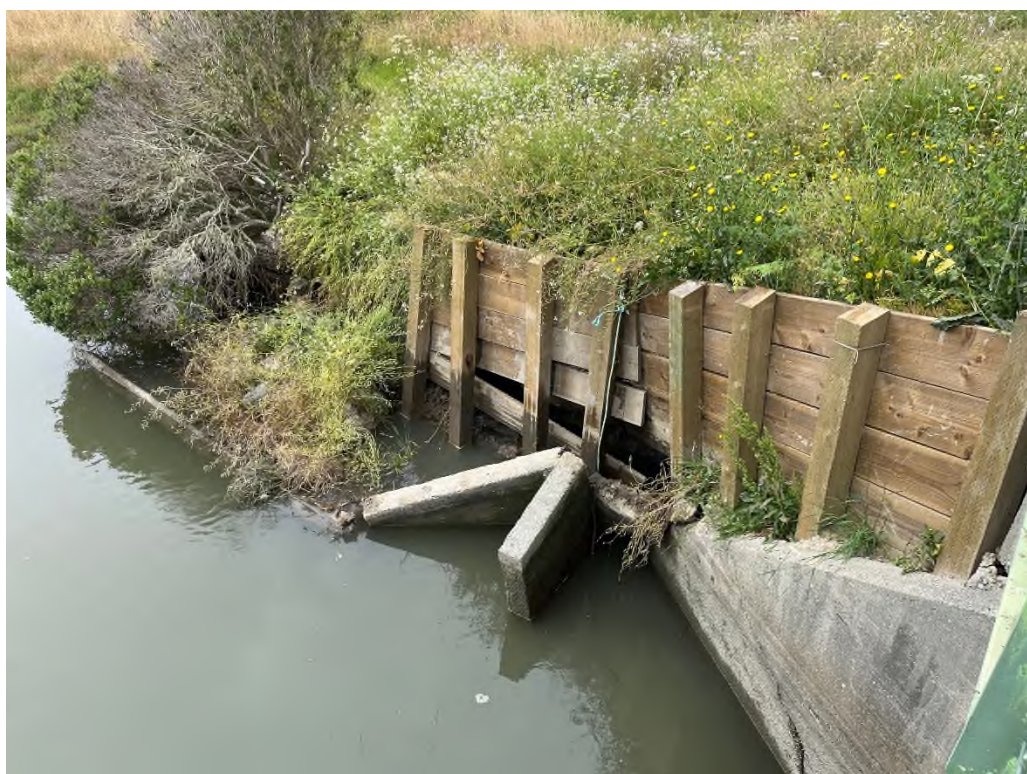
Photo 4: Further damage to South wingwall
