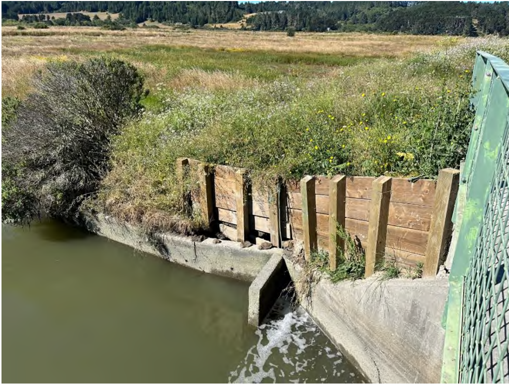
Photo 1: South wingwall, timber retaining wall, and evidence of water seepage
